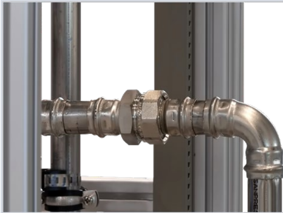
Figure 4: Connect the lower pipe union
